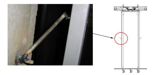
7、 Adjust the verticality of the door hanging board.center and header
